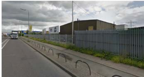
Photo 9 - View looking north west along Watermead Way, with the site to the left.
