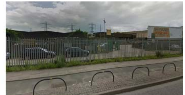
Photo 6 - View of the site along Watermead Way
