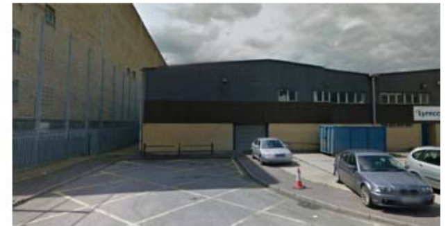
Photo 13 - View looking east from Leeside Road at southern end of the site, showing the current units on site.
